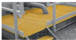
Raised work platforms
